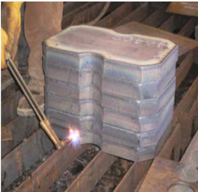
Figure 5. Manually post heating.
